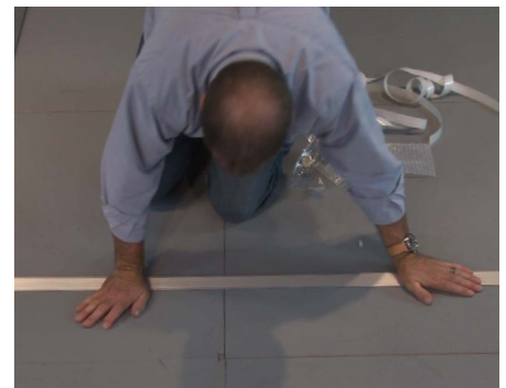
6 Firmly press down on the entire length of the frame to activate the tape.
