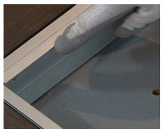
**3** The tread rails are at 1.5" on center increments. Filler bars may be required to achieve the exact overall dimension.
