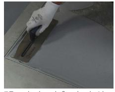
**7** To make the sub-floor level with the bottom frame leg, use non-shrink grout and trowel flush with the top of the bottom leg of the level base frame.
