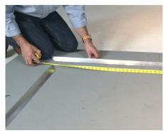
1 Dry fit all frame pieces within the area and use a tape measure to ensure a proper fit. For odd-shaped layouts, match frame tags to the drawing on the pack list.
