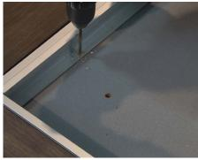
**5** Using a 5/32" masonry bit, drill into the concrete every 24" center. Fasten the frame with the supplied masonry anchors using a #2 Phillips-head screwdriver.
