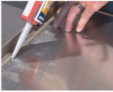
**12** Use silicone caulking to caulk the recess' perimeter seams and any seam where multiple pan sheets abut.
