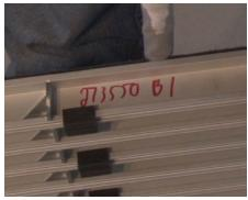
**13** Each grid module is labeled per the drawings to identify location. Begin placing modules in the recess per the shop drawing layout.
