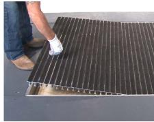
**20** Care & Maintenance: to clean beneath the grid, use a slotted screwdriver to remove grid. Place wood blocking under grid and remove panels.
