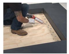
**10** Proceed to the drain pan installation. Use a caulk gun to apply adhesive on top of the newly grouted area.
