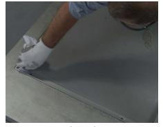
**9** Use a rag to clean the excess grouting from the top of the frame leg. Allow 24 hours for the grout to dry before continuing with the installation.
