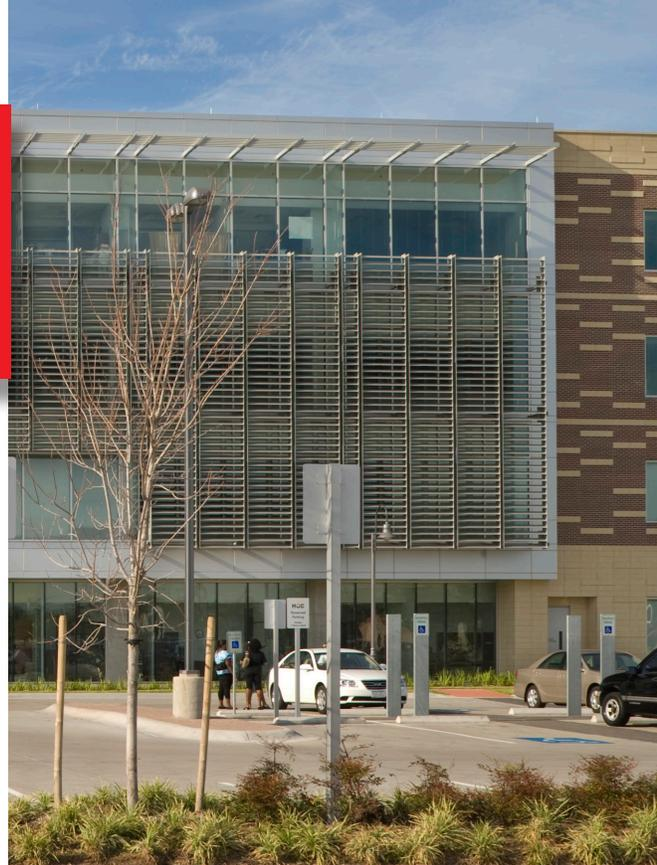
C/S Fixed Horizontal Sunshades make a dramatic statement and significantly reduce the interior heat and glare at HCC. HOK specified a custom horizontal “ladder type” airfoil sunshade to control the morning and afternoon sun that affects both the front and atrium portions of the building. The exposed mullions attached to the masonry walls are exaggerated to add drama to the sunshade design.
