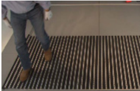
3. Align the mat into the recess.
